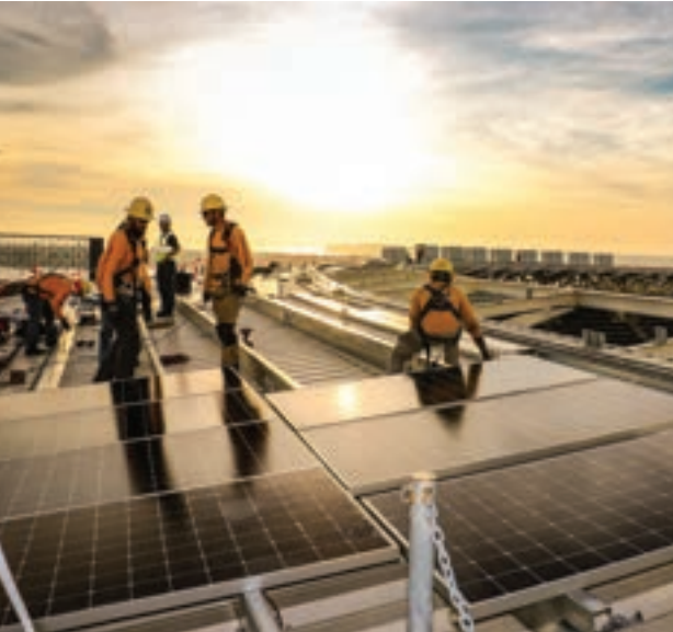
Turnkey Project (SITC), Solar
