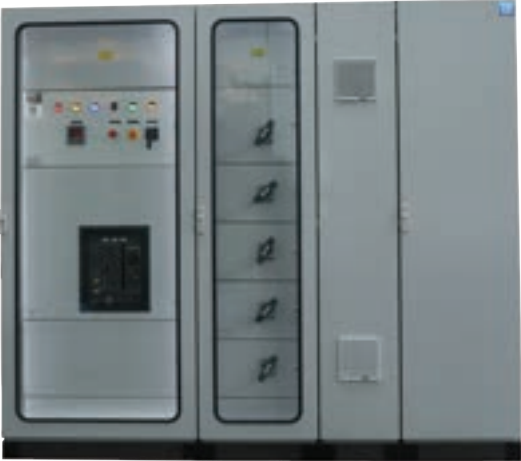
Solar Power Panel
